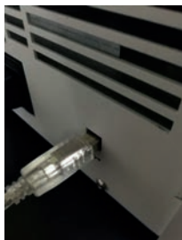
Inconsistent data cable
